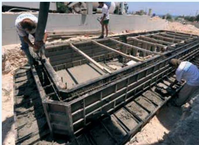
A full 20cm thick concrete wall with footing is erected.
