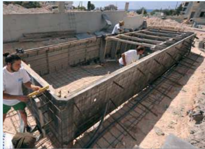
Saratoga aluminium wall forms are erected, and steel reinforcement is placed.
