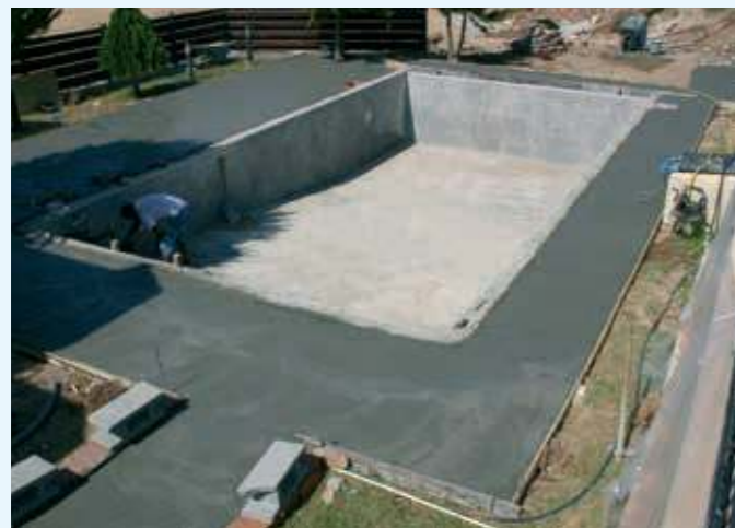
Reinforced concrete is placed around the pool.
