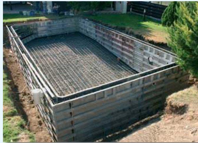
Saratoga aluminium wall forms are erected.
