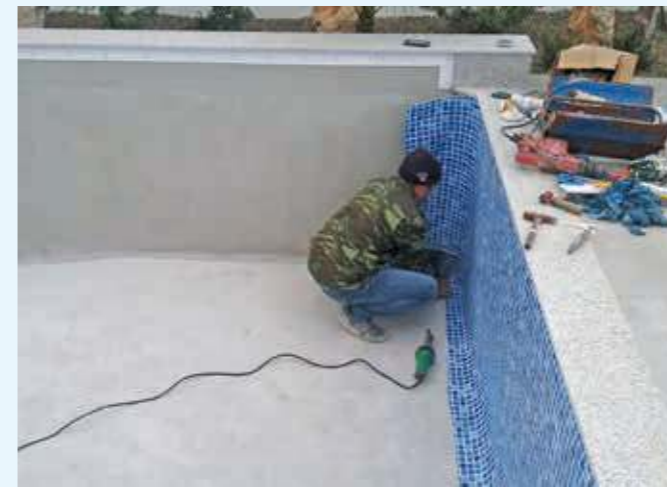
The PVC Membrane is secured into the bead receptor, turning the super-structure into a beautiful, virtually maintenance free interior surface, firm and smooth to the touch.
