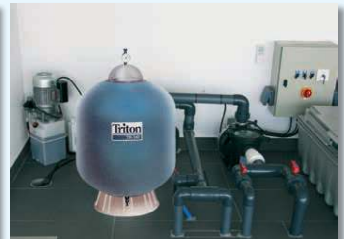
Installation of the pool's filtration.
