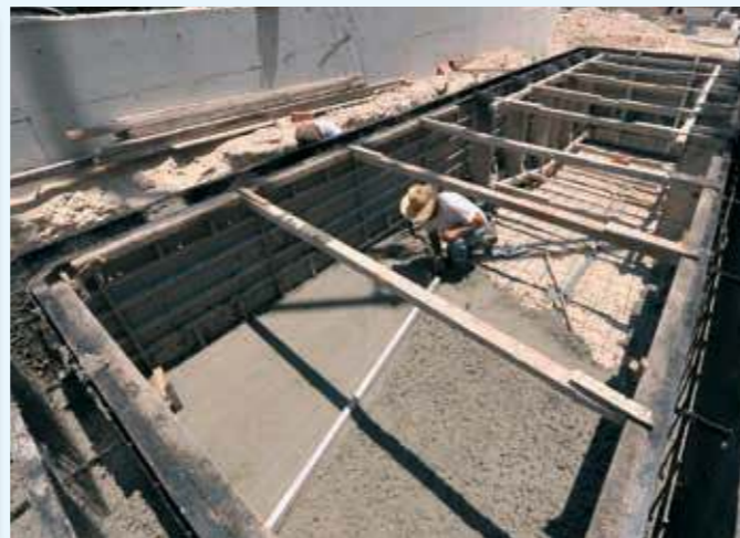
A concrete screed is poured in the pool bottom.
