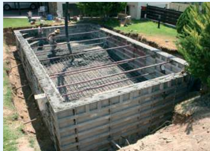
A thick reinforced concrete screed is poured in the pool bottom.
