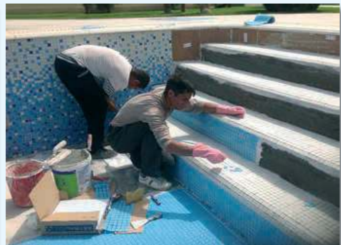
A professional worker places ceramic tiles on a SARATOGA pool wall.
