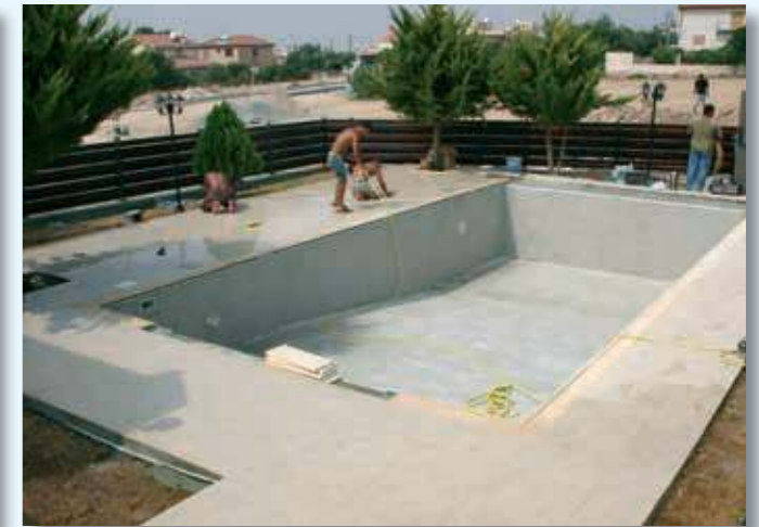
Installation of the patio around the pool.
